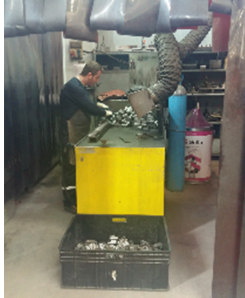
GAS WELDING TABLE 1.2 mm Wire / 320- 500 A ARCTECH (3 pcs) GEDİK FRONIUS (1 pcs) EXPRESS WELD (1 pcs) TURALLAR (2 pcs) DAIHEN (1 pcs)
